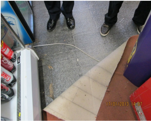
2) Cables trailing across walkways and under carpet and consumer units behind refrigeration.
